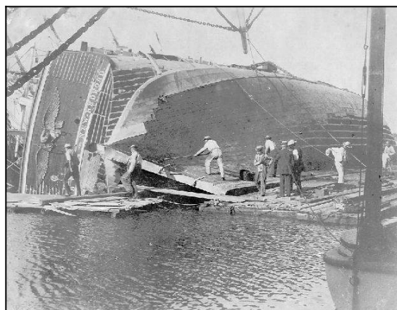
SUNBEAM hove down with crew hard at work (NB Whaling Museum Photo)
