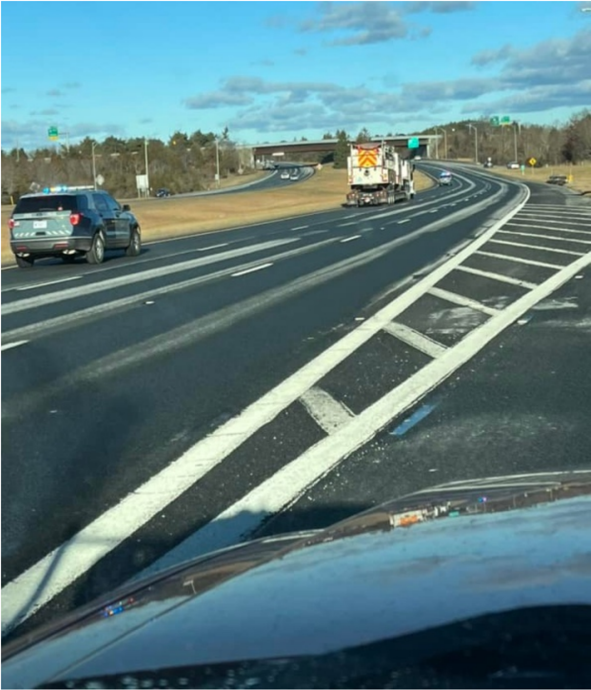
Rochester Fire Department photo.
