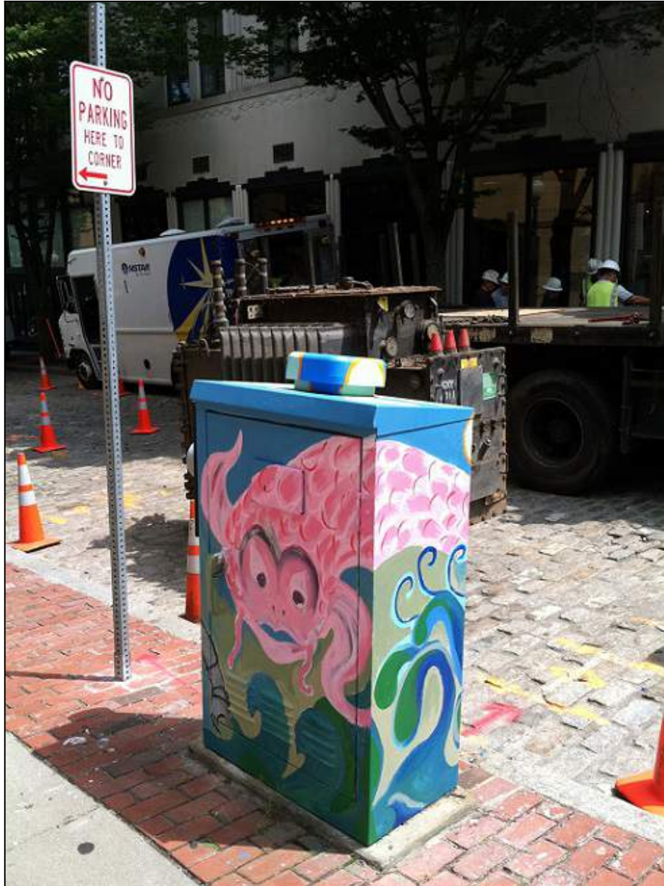
One of the finished commissioned electrical boxes
