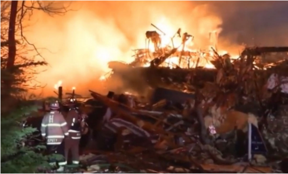
Truro Fire Department photo.
