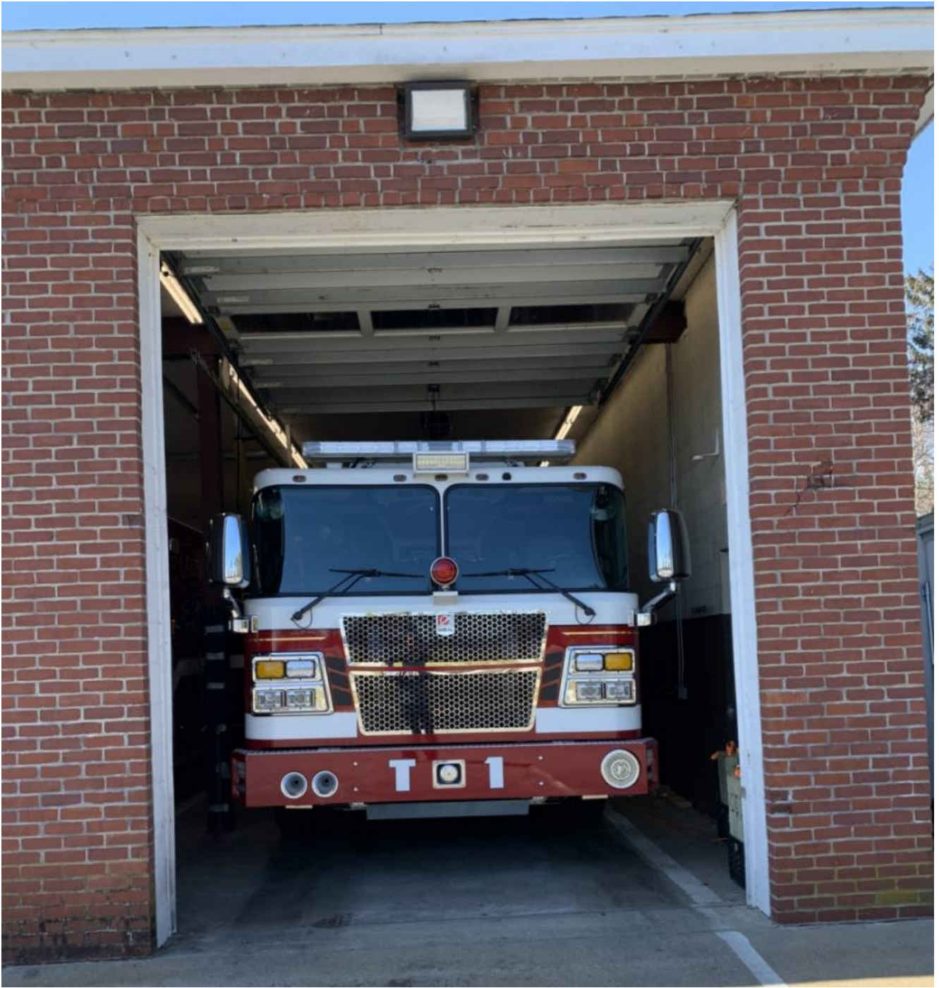
Lakeville Fire Department photo.
